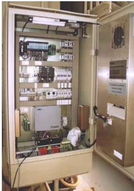
PD Monitoring System installed on the busbar of a turbo generator
